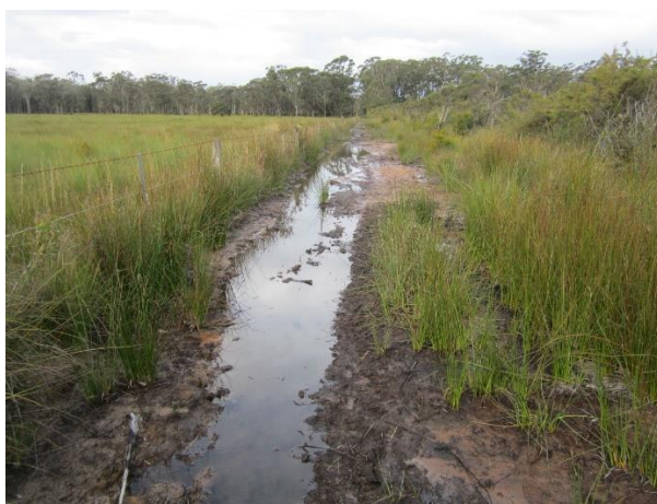
18/9/2015 - Surface water in poorly drained area on northern site boundary. Peat soils exposed by service trenching works.
