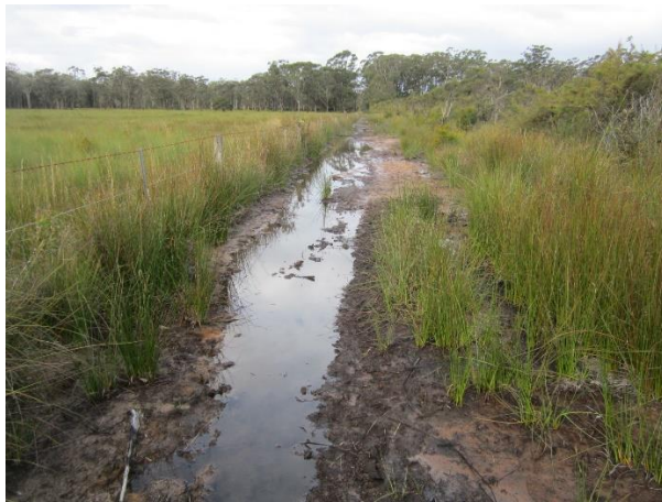
Surface water in poorly drained area on northern site boundary. Peat soils exposed by service trenching works.
