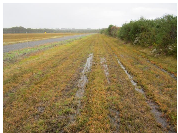
Grass access track adjacent to runway area. Water pooling in wheel tracks.
