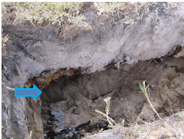
TP2 – Typical profile with aeolian sands, overlying a thin upper indurated sand horizon, overlying more aeolian sands. The test pit is collapsing due to water inflow occurring above a lower indurated sand layer (not visible).
